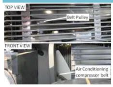
**Details** Air conditioner compressor belt pulley.
